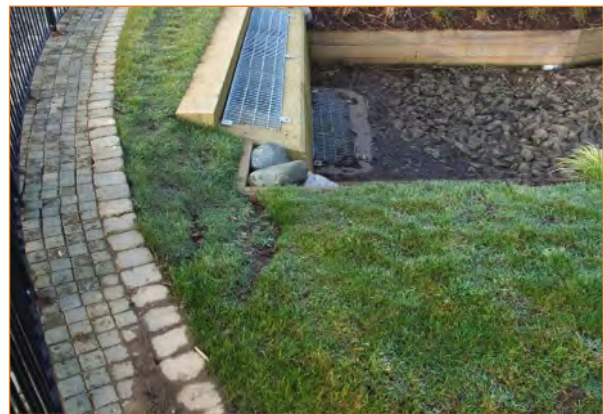
Figure 14.20: Swales at Upton, Northampton, UK
