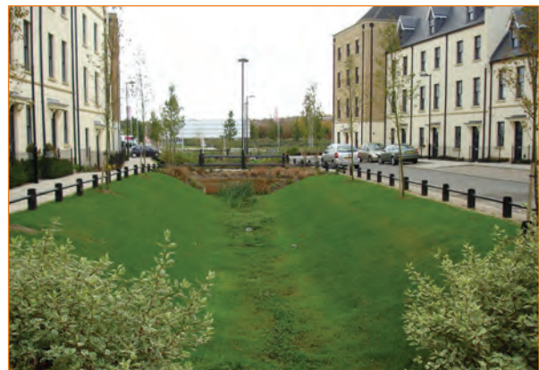
Figure 14.19: Swales at Upton, Northampton, UK
